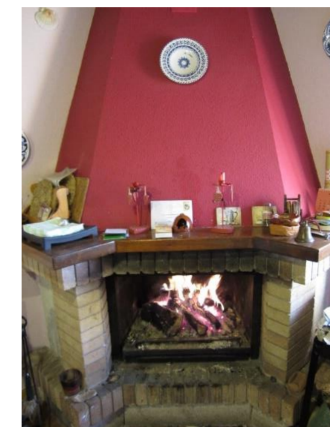
Fig. 3. Open fireplace with a combustion chamber volume of 0.09 m 3 , corresponding to 0.35 m height, with a trapezoidal base of 0.52, and 0.63 m width and 0.45 m depth. The room volume was 41 m 3
